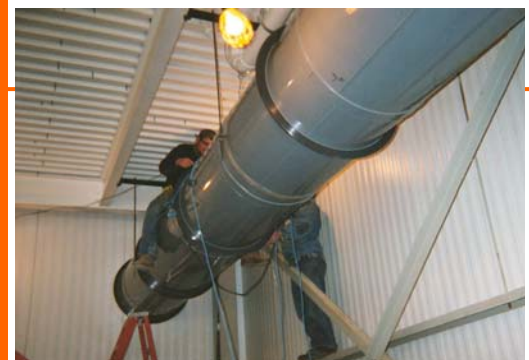
CORZAN™ CPVC DUCT INSTALLATION
